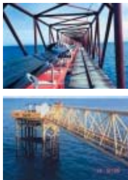
New construction of conveyor belt
