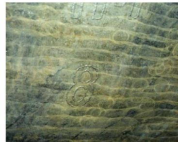
In addition steel, with active corrosion pitting, shows a mottled appearance after hydro blasting. Mottling occurs when the corrosion products are washed out of the pits, leaving a bright patch, and the surrounding areas are left a dull grey, brown to black colour. This pattern is the reverse of that left by abrasive blasting, where anodic pits are often dark, due to corrosion products not being entirely removed, and the surrounding areas are bright.
